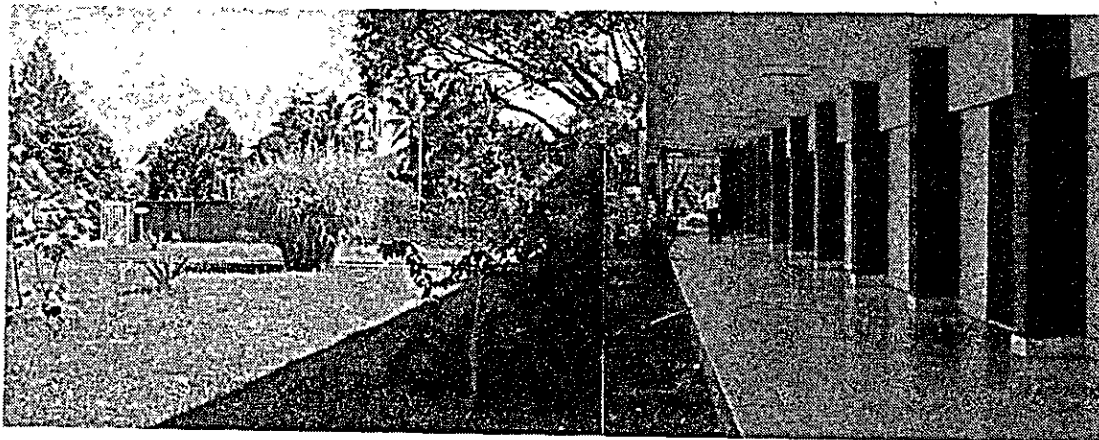
A building of Parapat telephone exchange, which is modern and accomodates the cross-bar type automatic exchange.
