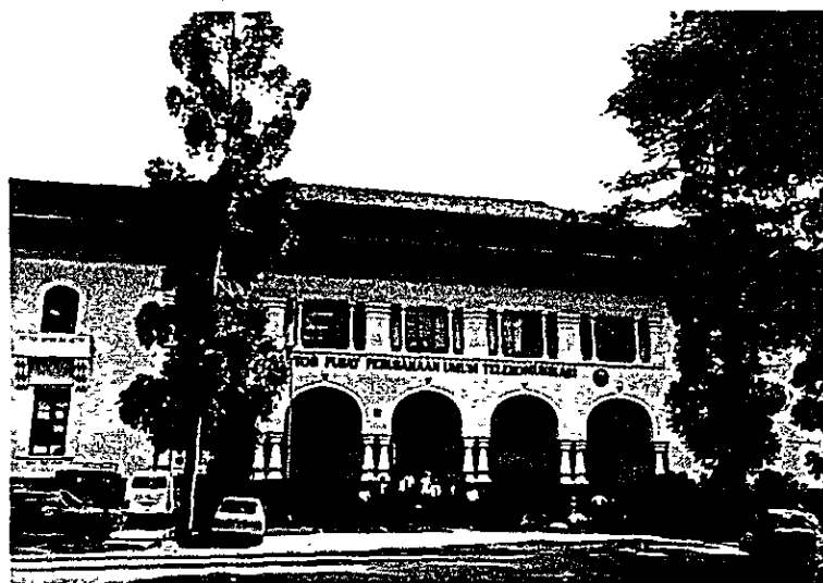
Front view of the PERUMTEL Head Office, an attractively designed building which harmonizes with the surrounding landscape
