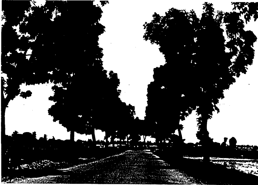
A view of existing road in the improvement section
