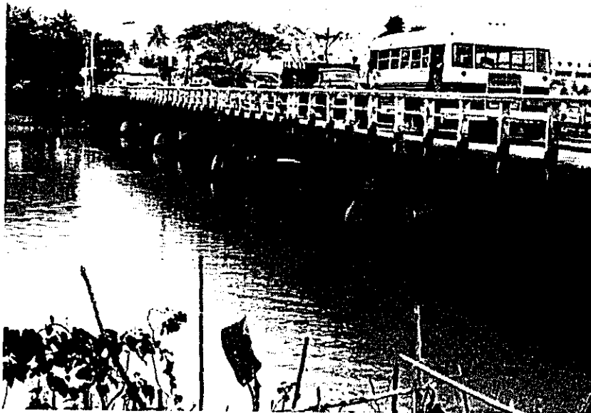
Existing Ci Sadane bridge: The Tangerang city develops centering around Ci Sadane river
