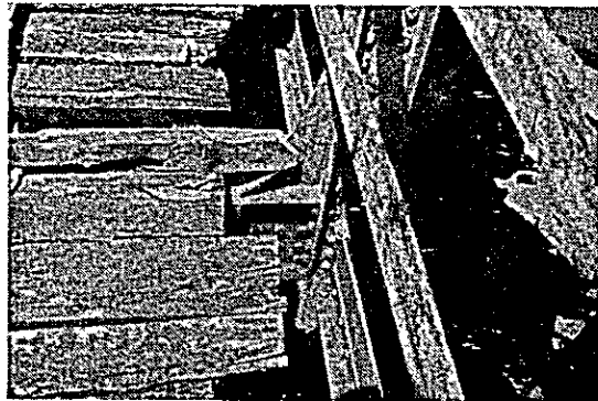
Girder portion of Sarambu bridge, 339.8 km from Makassar.
