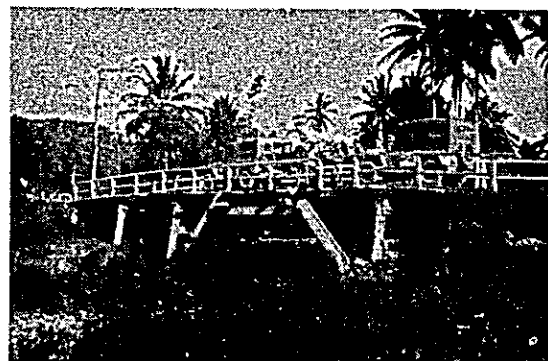
Muntoi wooden bridge 13.7 km from Kotamobagu
