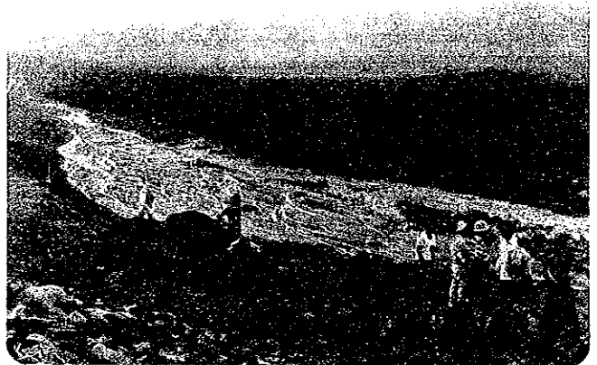
Photo-24 Besuk Sat Lama Overtopping occurred because of small passing capacity due to narrow width of the channel. Revetment work was completed in order to prevent a flood to Lumajang. But flooded. This part must be widen urgently.
