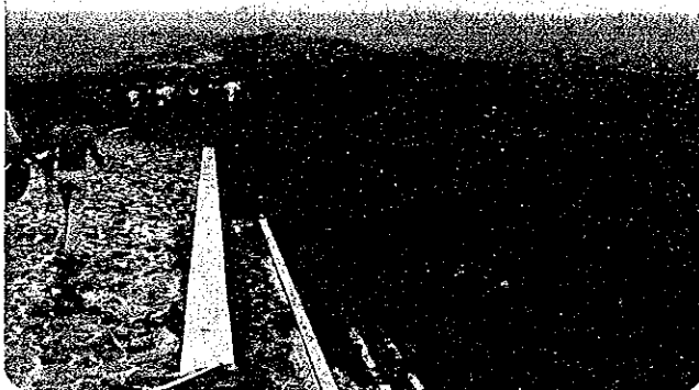
Photo-21 Situation of Besuk Sat trunk river This photo shows that the dam checked the material to Lumajang effectively and regulated the flow effectively.
