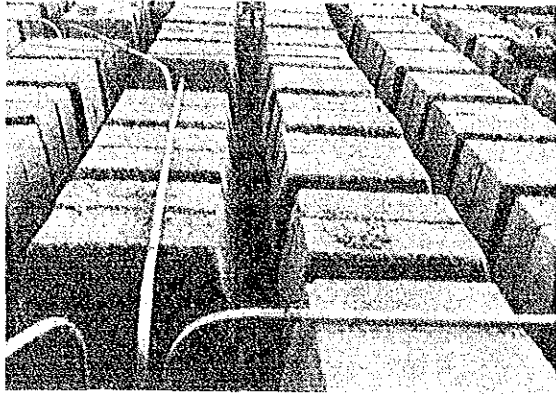
Joist slab method using floor blocks
