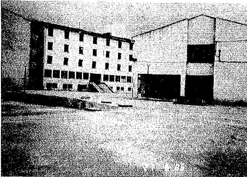
〔 Tuzla Vocational High School の本館と学生寮 〕
