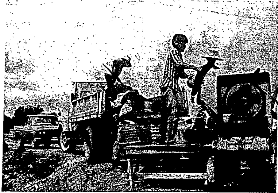
Putting materials into the mixer
