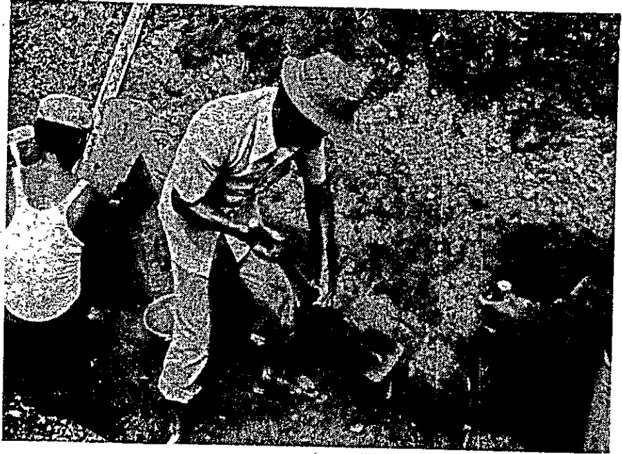
Compaction by a hoe and finishing of surface by a wooden flation
