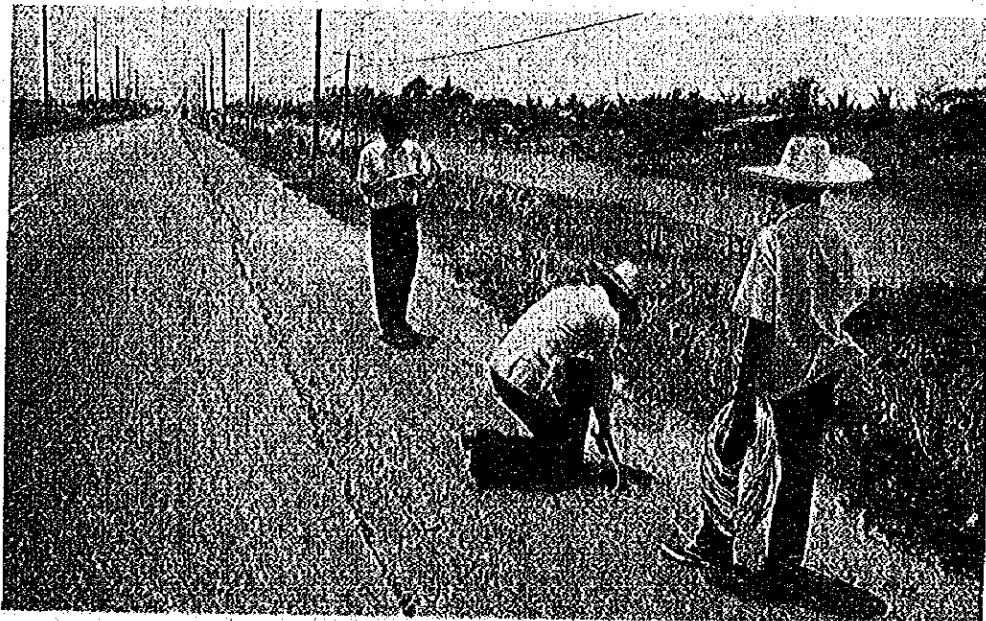
2. Survey of Aerial Route between SPK and BPO Exchanges.
