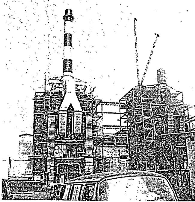
Photo. 3-3 South Bangkok Thermal Power Plant Under Construction
