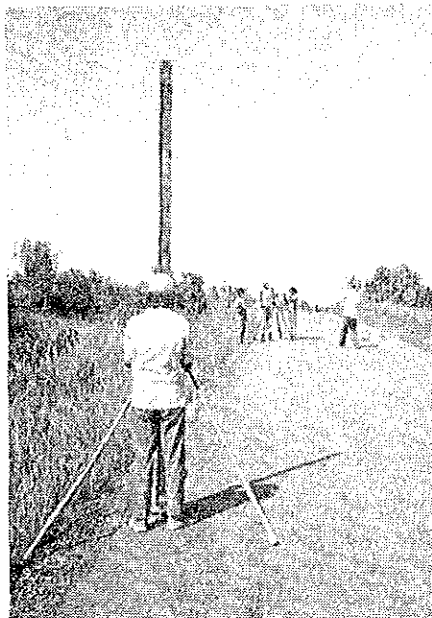
Second order levelling on the flat section of the route (mostly undulated)
