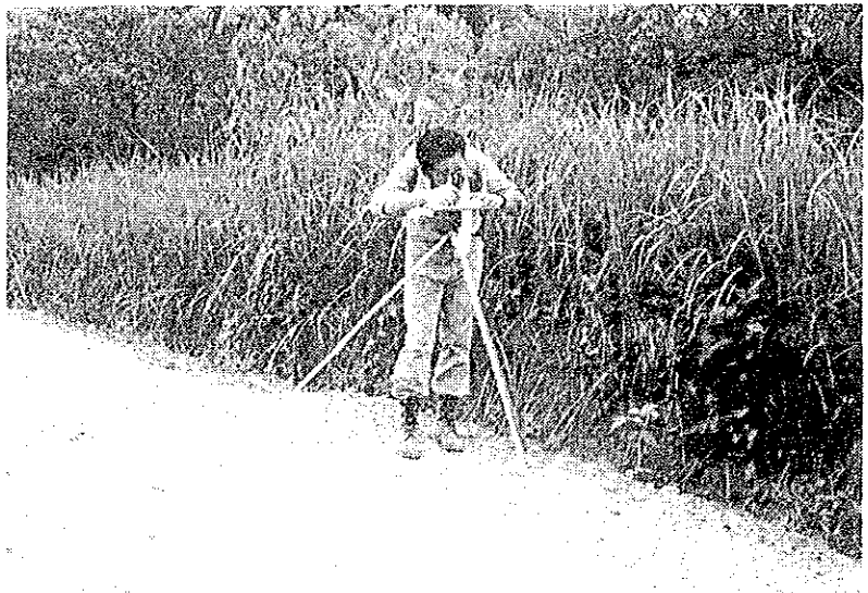
Field Completion (Plane table survey on newly constructed highway connecting Tanjung and Murungpudak)
