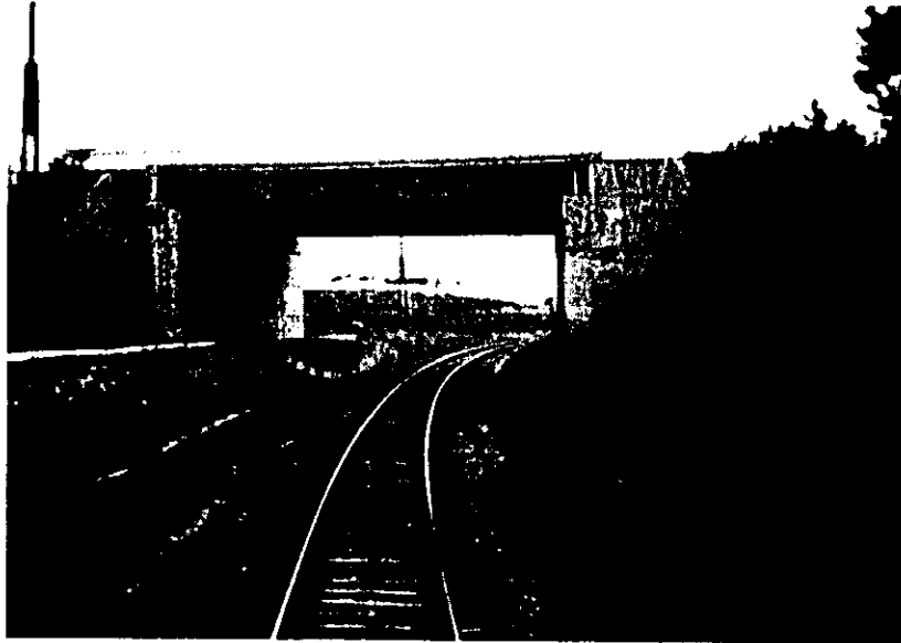
Mi Ho ~ Jeong Bong (Near 9.6 km Point) (R = 400 m)
