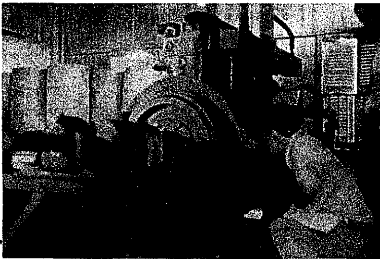
Generator at Mimot
