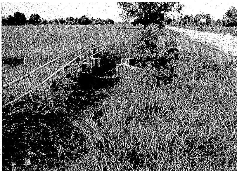
(16) Paddy fields to be irrigated (left side) and existing water delivery system (centre). The latter is not operational due to lack of pumping capacity.
