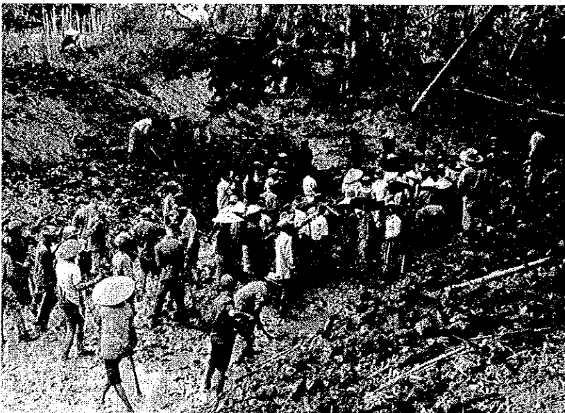
4. Enlargement of channel with hand labour
