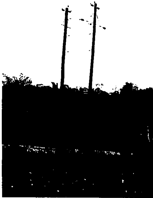
H Pole (Crossing of River 200m) at Jones
