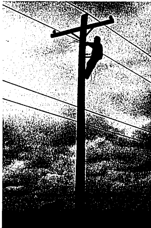
Construction Work of Distribution Line at Jones Line (ISELCO)
