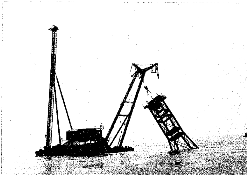
The inclined boring tower by the strong tidal current at Shoal-A.
