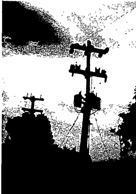
Aerial electric lines in service for FAC
