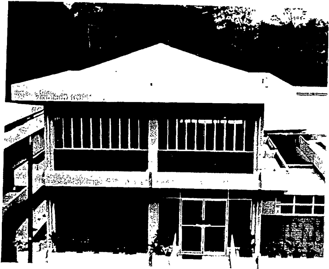
Office of the Project Leader (down) & Conference Room (up)
