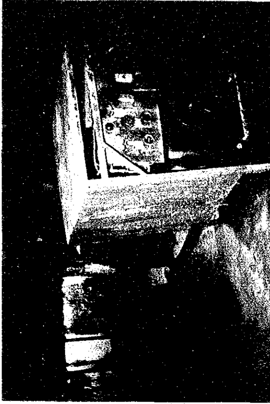
Not-working Actuator unit of EDF Damper under operation Control Arm
