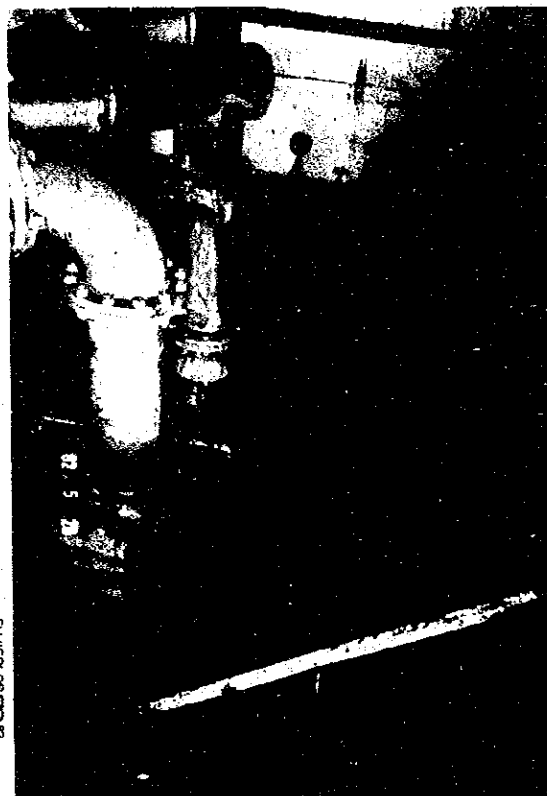
Malaya Thermal Power Plant Unit No. 1, 2 Ash Handling Slurry pump
