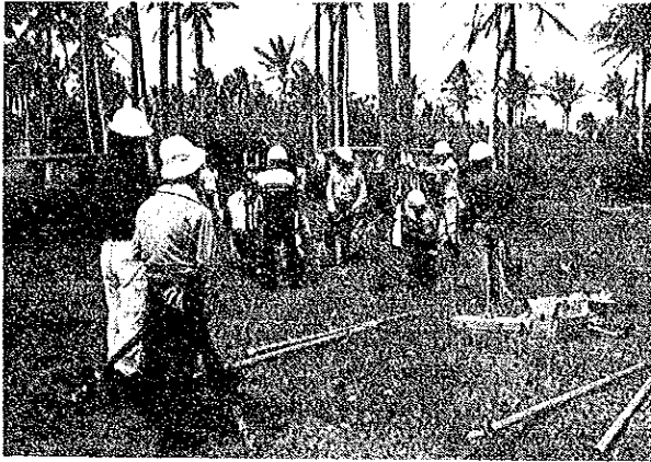
Foundation Work for Erection of Observation Tower
