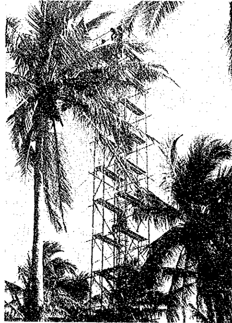
Erected Observation Tower (approx. 24m high)
