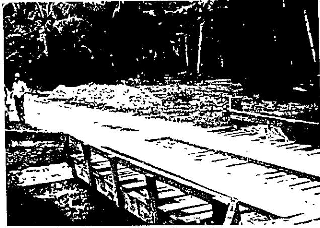
(28) Highway and bridge near Remery
