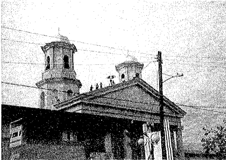
Observation at newly established control point on the roof of Malabon Church
