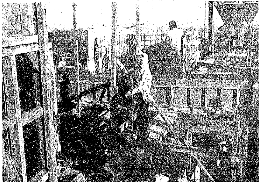
Erection of Forms
