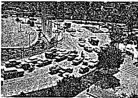
Fig. 5-2-13 Traffic lights provided at each inlet of rotary also stop vehicles circling around the rotary
