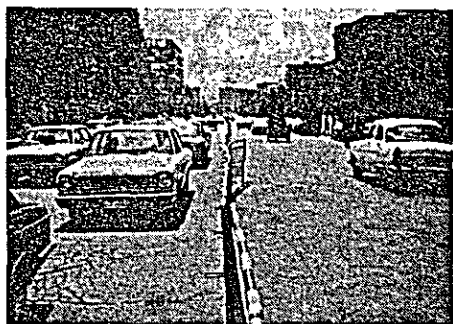
Fig. 5-2-9 Alignment of fence is disrupted by pedestrians trying to cross the road at undesignated location.
