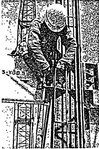
Photo 6: jointing of beam to a column
