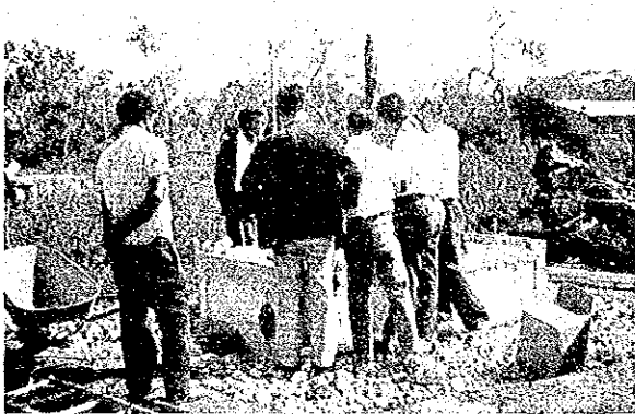
WHO Urban-Sewage and Drainage Project (septic tanks)
