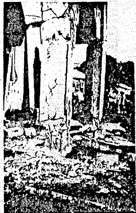
FIGURE 25: COLUMNS SUPPORTING TOWER FREE WESLEYAN CHURCH, PETANI, 'EUA
