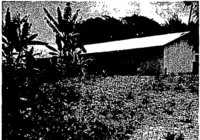
(Existing Facilities: Kira Kira)
