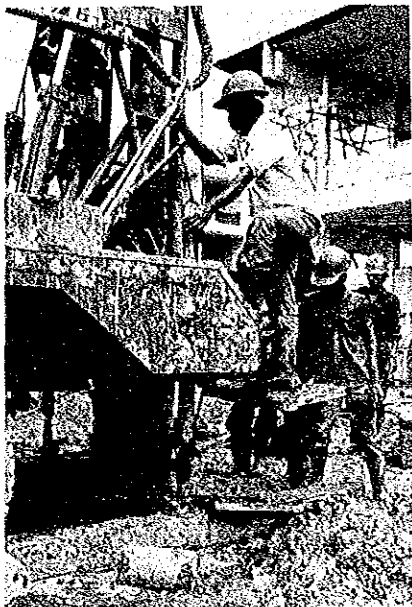
A view of auger drilling for cast-in-place pile (MAAD YAI Provincial Hospital )
