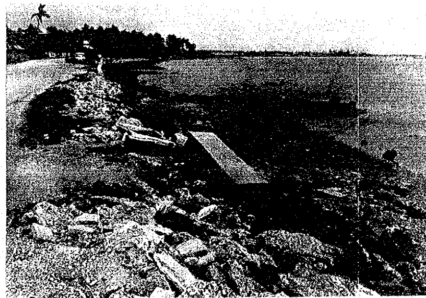
Existing Condition of Parapet (Eastern Seashore)
