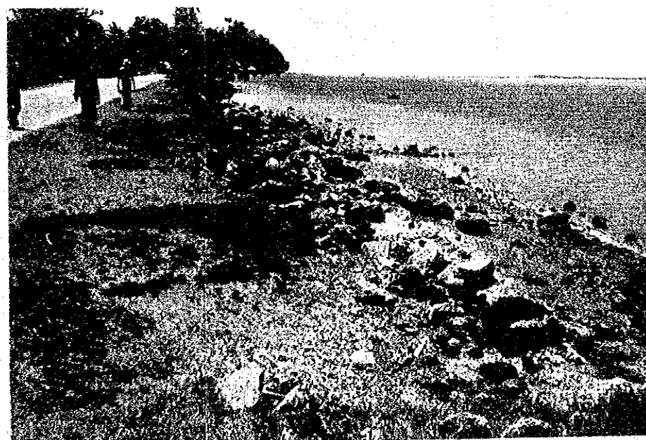
Damadge of Stone Masonry (Western Seashore)
