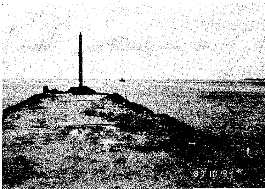
Existing jetty in Melekeok Harbor
