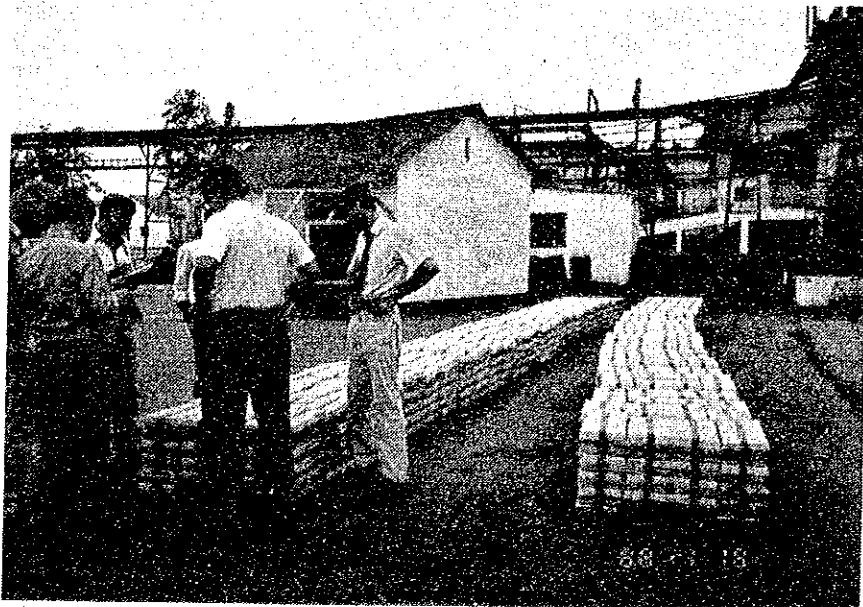
Sable 2 Zinc, Kabwe Plant
