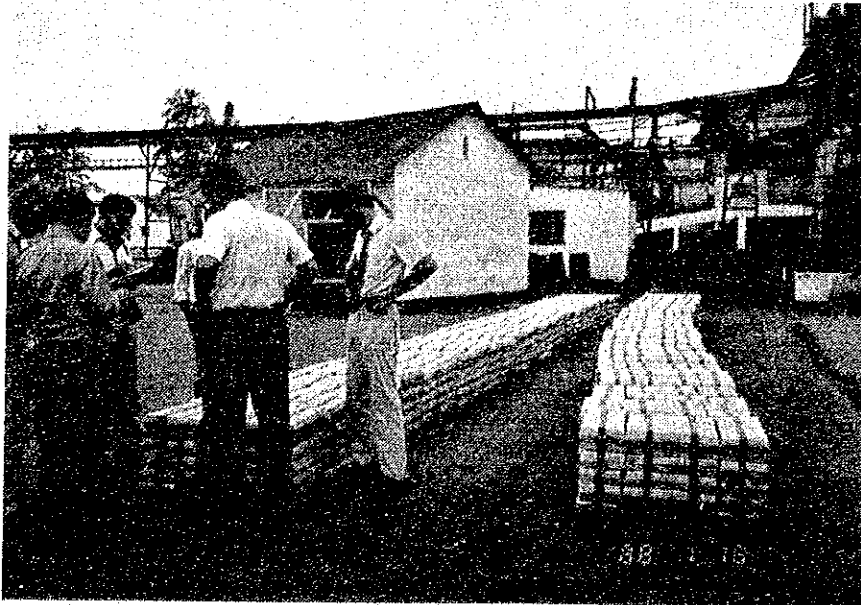
Sable 2 Zinc, Kabwe Plant
