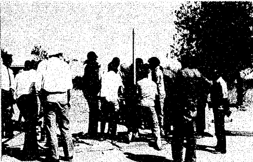
Villagers helping to repair a borehole pump in the Livulezi Project Area
