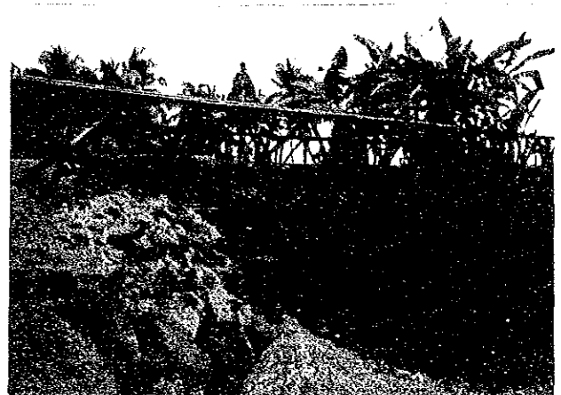
NAME OF BRIDGE : DANGOLAN BRIDGE
