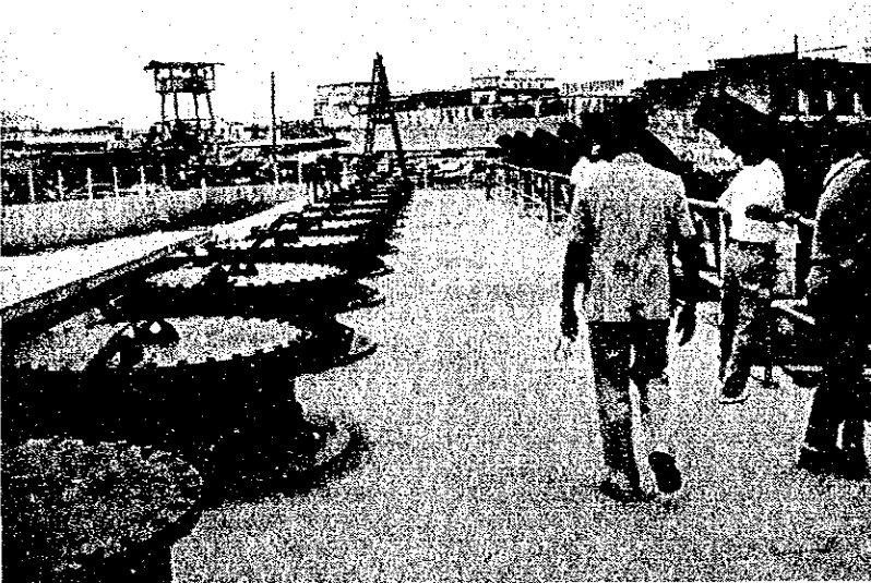
Installation state of pumps and screens
