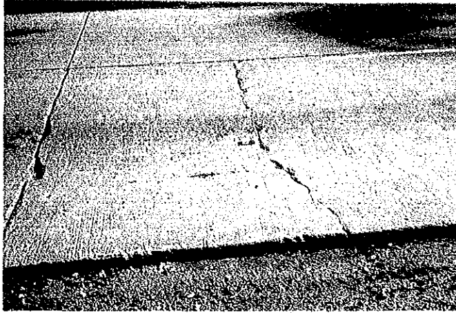
TRANSVERSE CRACK
