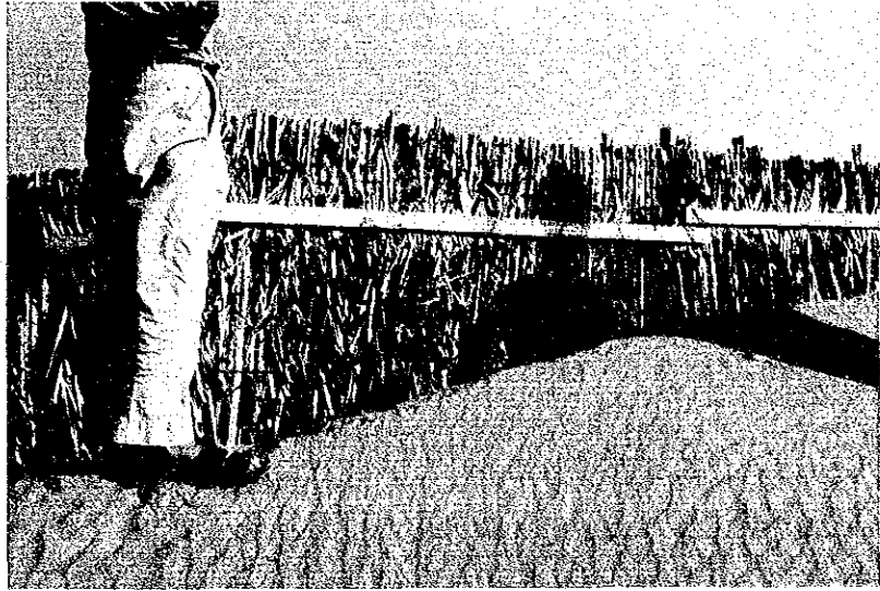
Construction of the sand fence by using Dates-fronds mat which made in U.S. E. – theme A.
