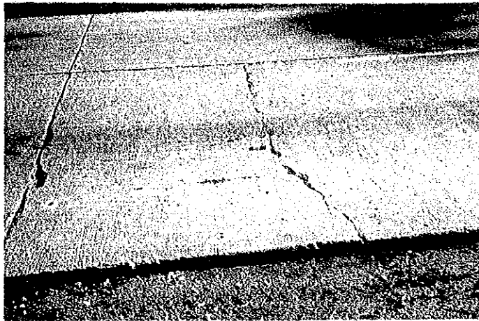
TRANSVERSE CRACK
