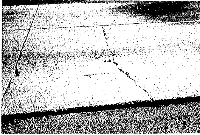
TRANSVERSE CRACK
