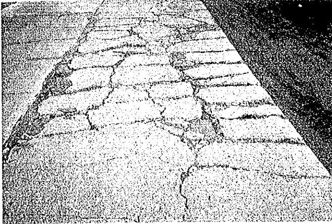
BLOCK CRACKING (Separation of Slab)
