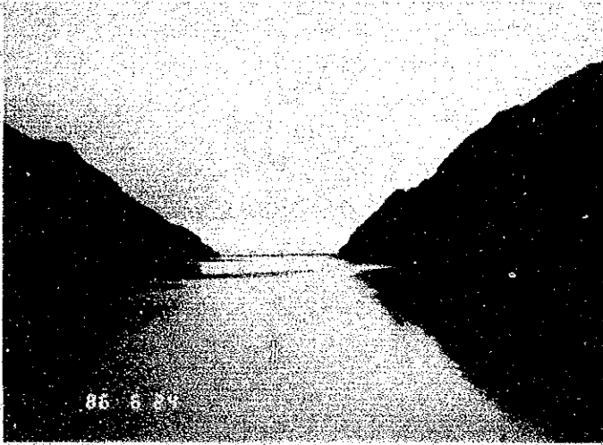
Distant view of Banaoang damsite, from upstream side (ID No.1-022-00-01-0)
