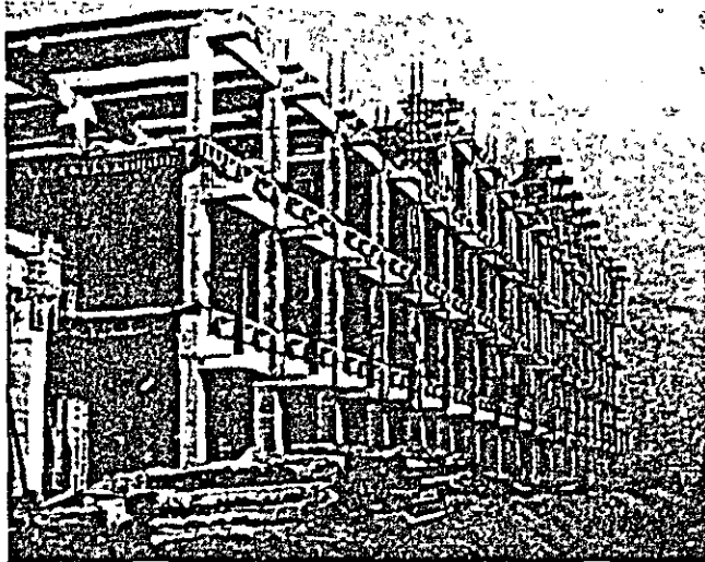
Photo 4.1 Industrial plant employing precast construction.
