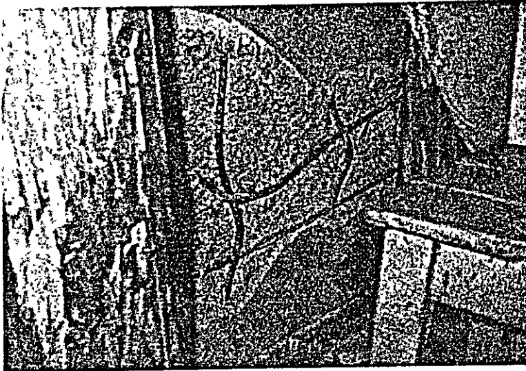
Photo 5.71 Failure of a 1st story wall in the span direction and buckling of reinforcing bars of a building of similar type, Bucharest.
