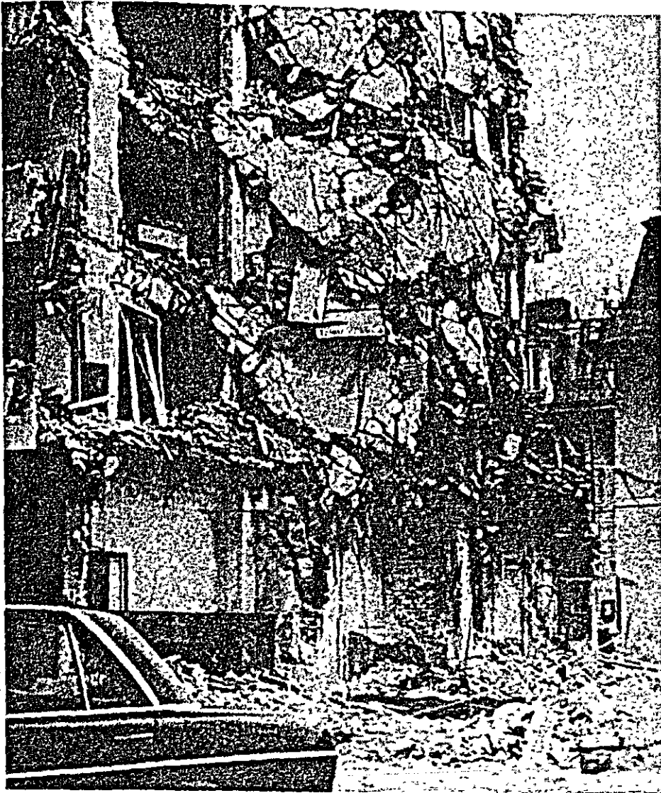
Photo 5.25 A destroyed building of reinforced brick construction No. 7, Bucharest.
