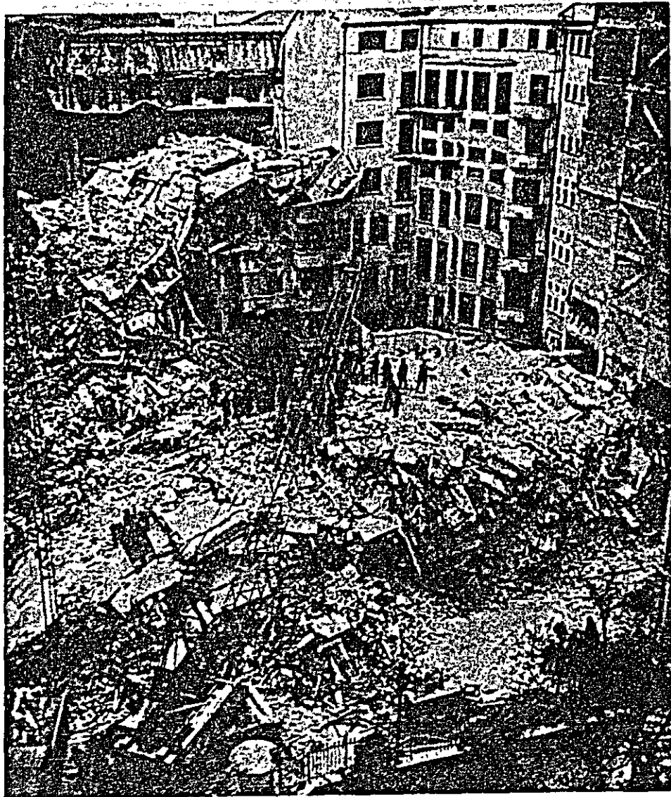
Photo 5.24 A fallen building of reinforced brick construction No. 6, Bucharest:
