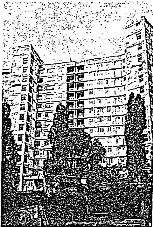
Photo 5.34 A 13-story apartment building of reinforced concrete rigid frame construction, Bucharest. (Non-structural walls are non-reinforced brick or block walls.)
