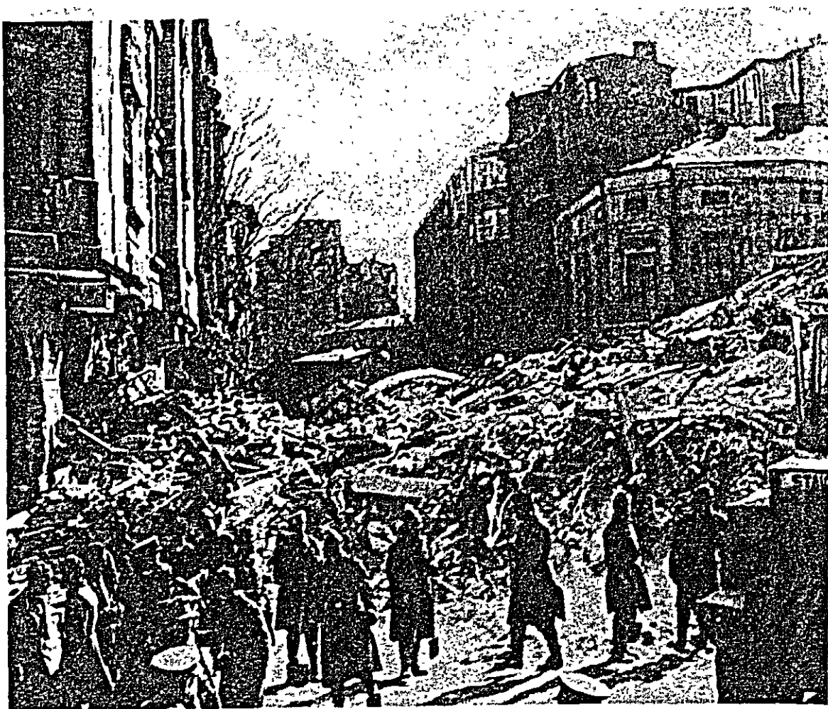
Photo 5.26 A destroyed building of reinforced brick construction No. 8, Bucharest.
