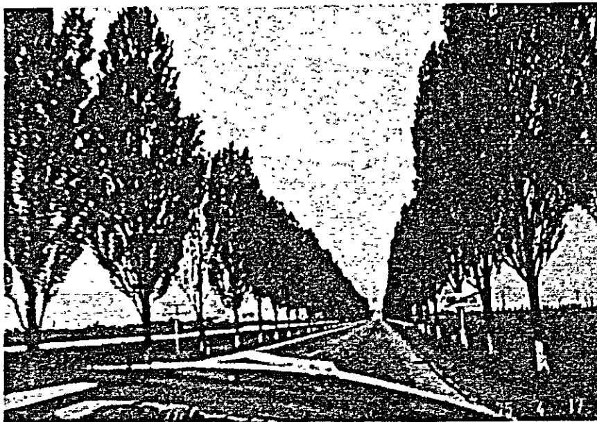
Photo 6.2 A national highway (Pitesti-Craiova)
