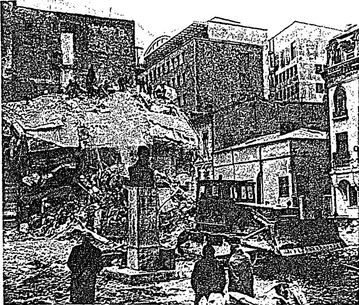
Photo 5.23 A collapsed building of reinforced brick construction No. 5, Bucharest.
