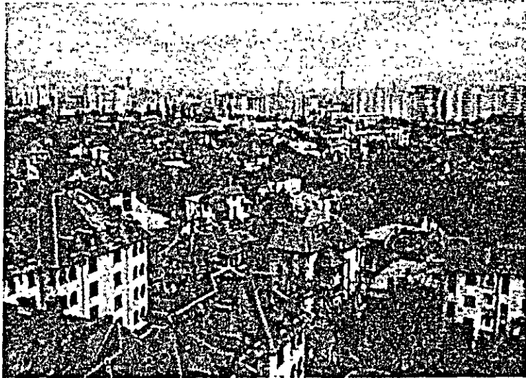
Photo 5.33 Panoramic view of Bucharest from the city center. (Buildings of brick or reinforced brick structures are in the foreground. Middle and high-story apartment houses in the distance are reinforced concrete buildings on the city's outskirts.)
