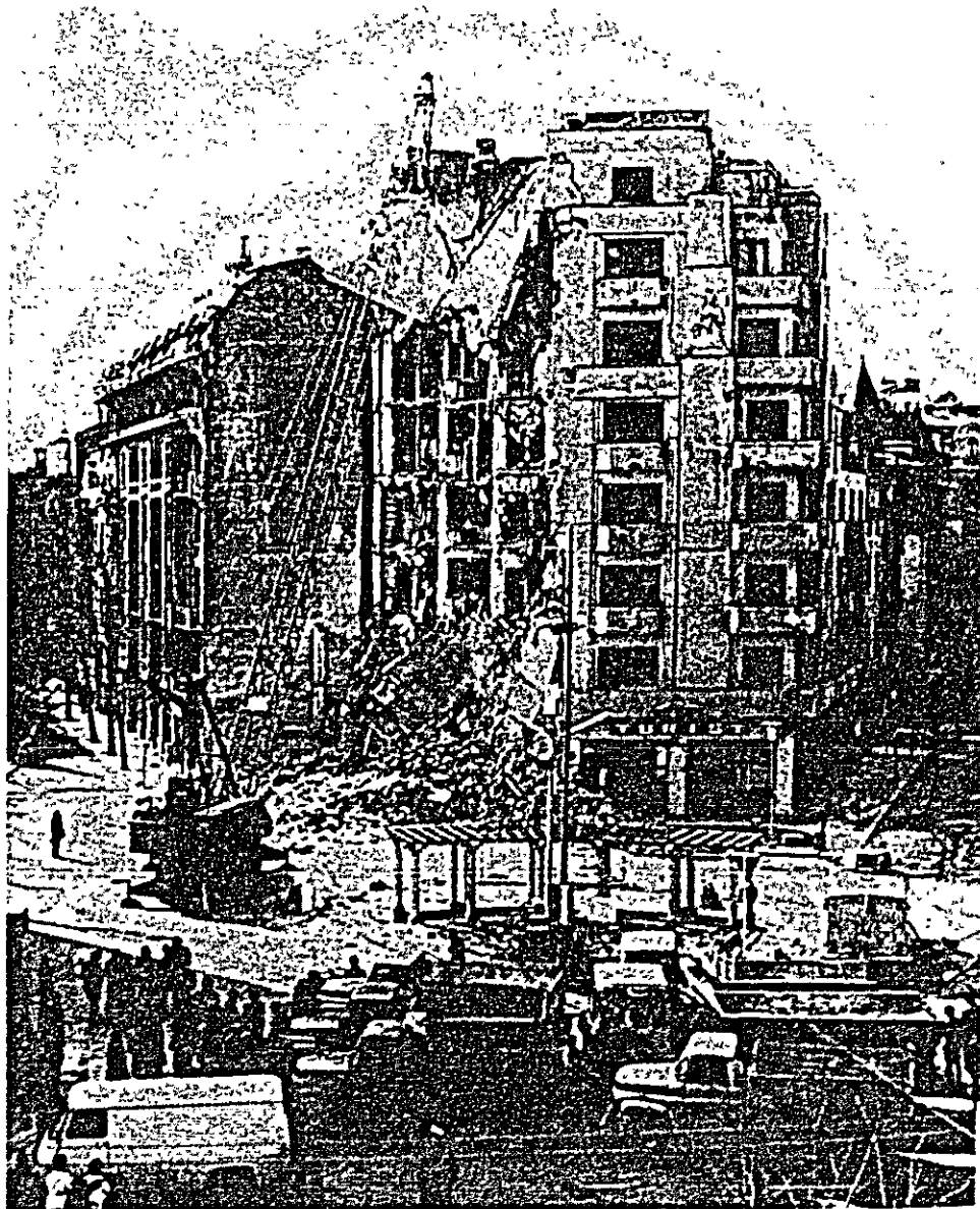
Photo 5.22 A destroyed building of reinforced brick construction No. 4, Bucharest.
