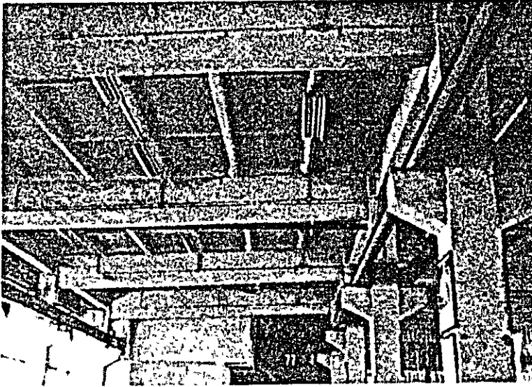
Photo 5.82 A five-story plant with cast-in-place rigid frame and precast floor slabs, Bucharest. (Slight damage to the structure)
