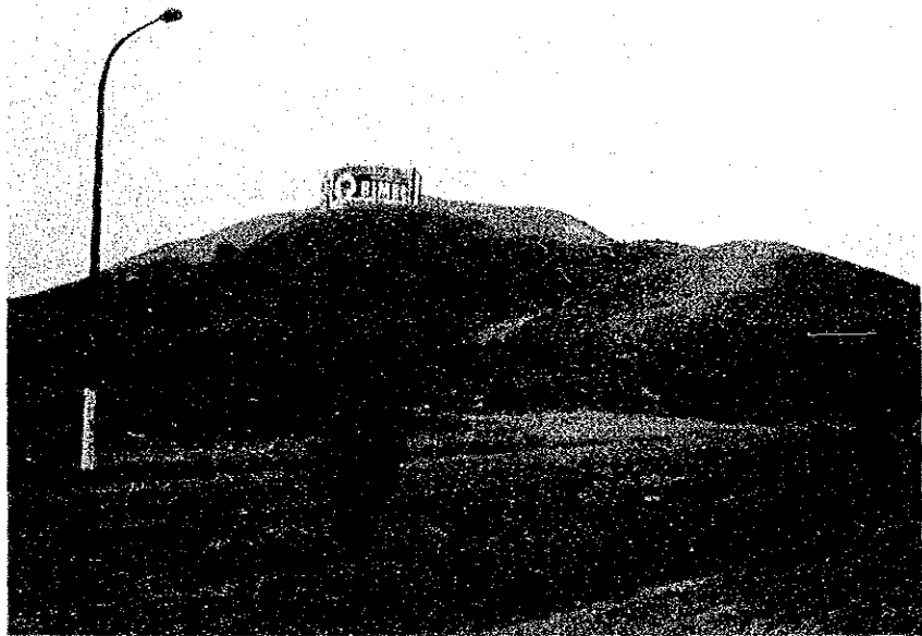
STORAGE RESERVOIR NO. 2
