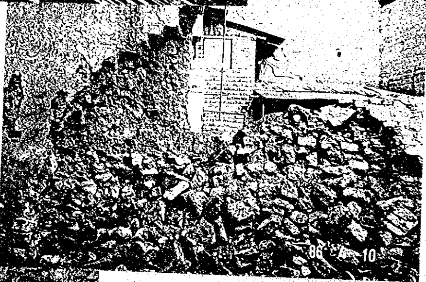
One of the adobe walls collapsed inside the building.
