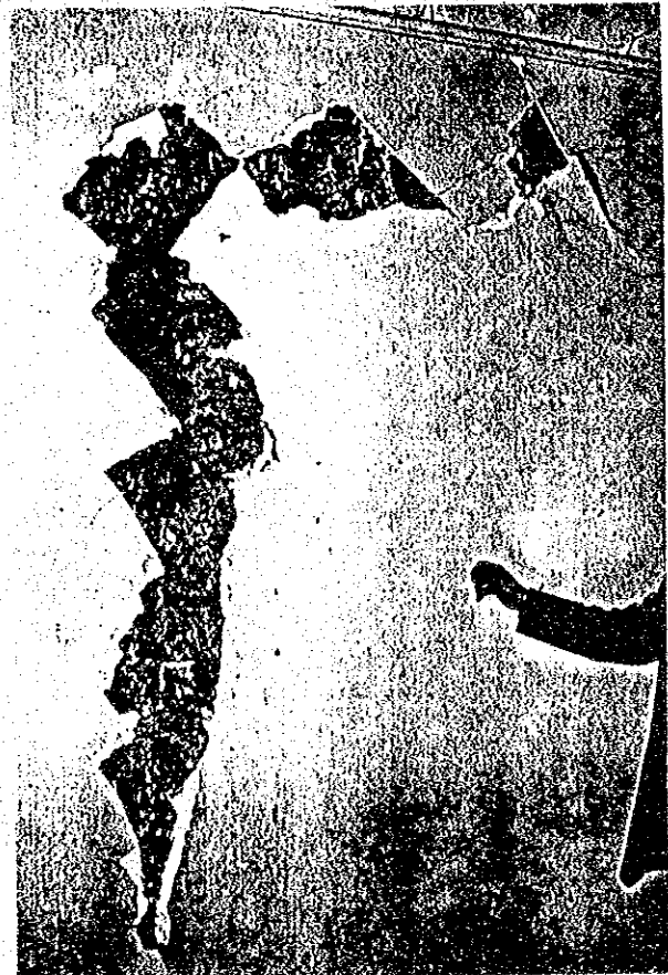
High school. This building is reinforced concrete frame structure; between the frame ordinary bricks are infilled. At the top floor (4th floor) bricks of corner wall were severely damaged. To prevent bricks from falling to the street, workers are destroying the brick wall.
