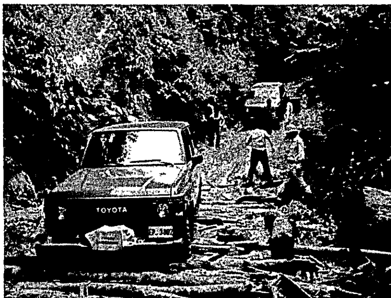
Repair of a road destroyed by landslide. It was seen everywhere in the survey area.
