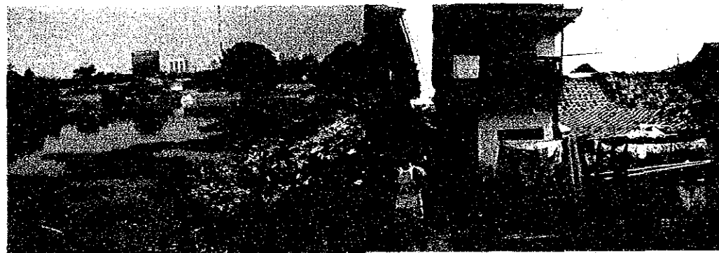
▲ PHOTO OF EXISTING CONDITION
