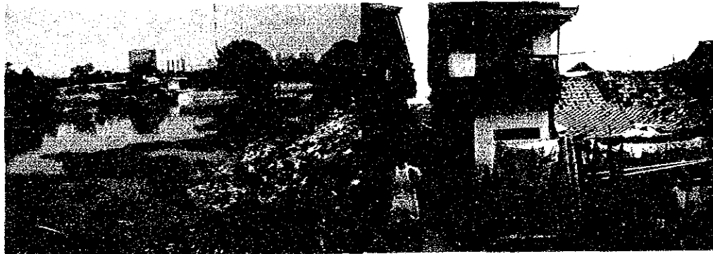
▲ PHOTO OF EXISTING CONDITION
