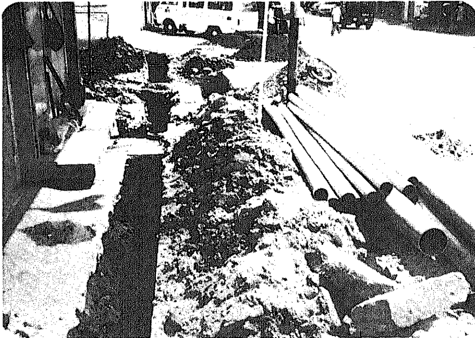
REPLACEMENT OF THE EXISTING DISTRIBUTION PIPELINE
